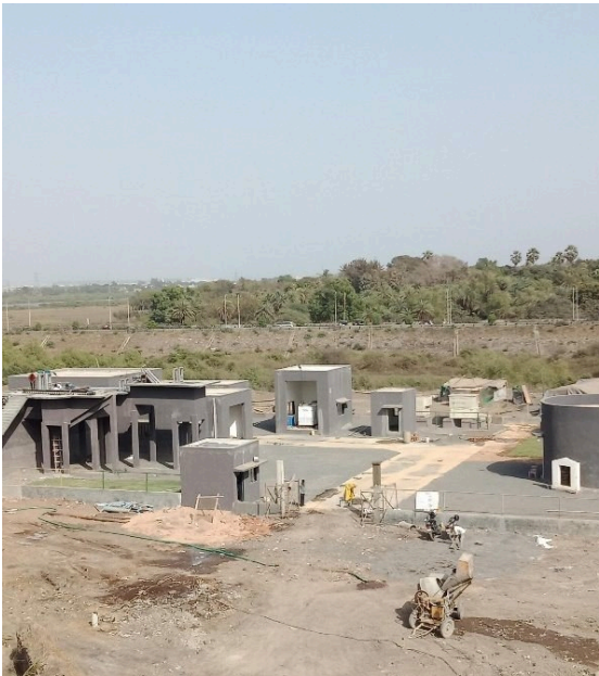
MUNICIPAL STP SITE — TANKS, BUILDINGS & ROADS
