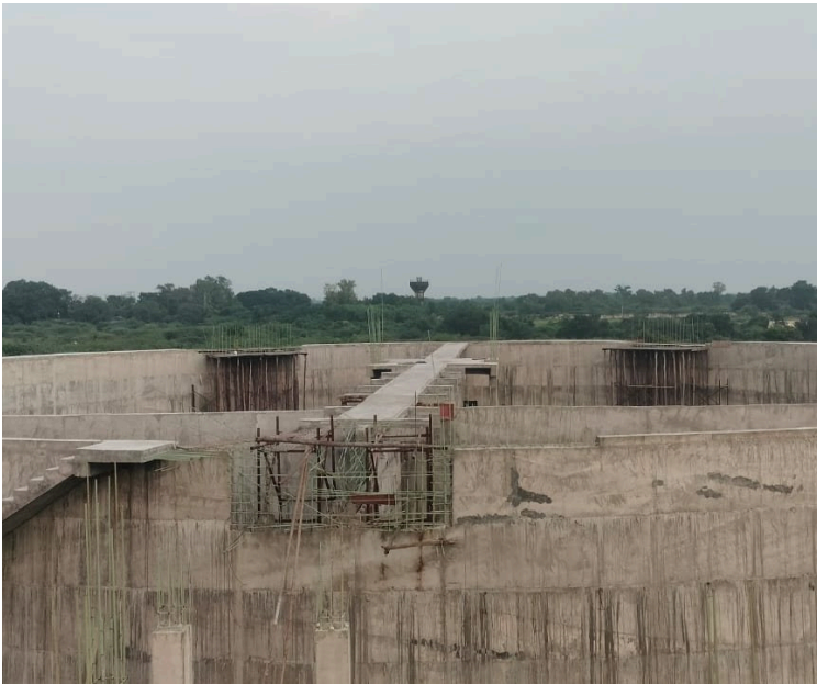
WATER-RETAINING STRUCTURE UNDER CONSTRUCTION
