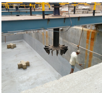
SURFACE AERATOR IN SERVICE
