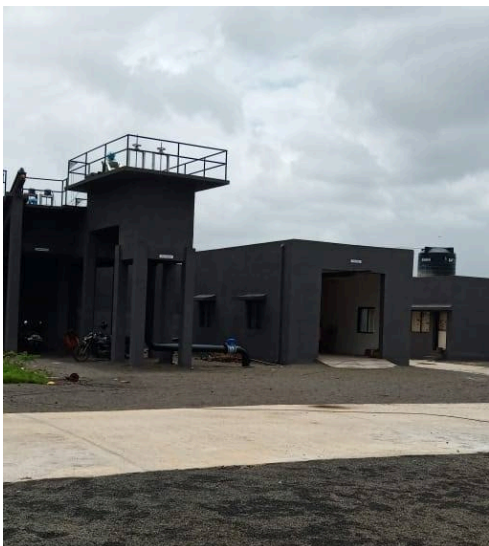
MUNICIPAL STP — CIVIL & STRUCTURAL WORKS
